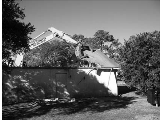
Demolition of the boathouse
